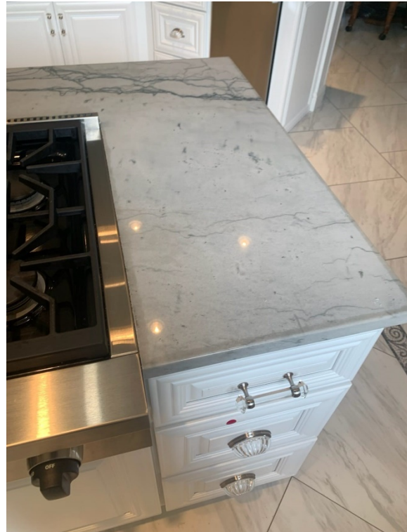
Fig. 3: Edge staining occurring after a few months
